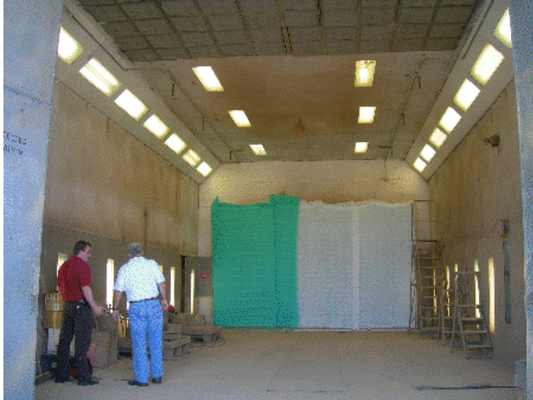
Figure 1. Overview of Building 9576 404th paint booth.
