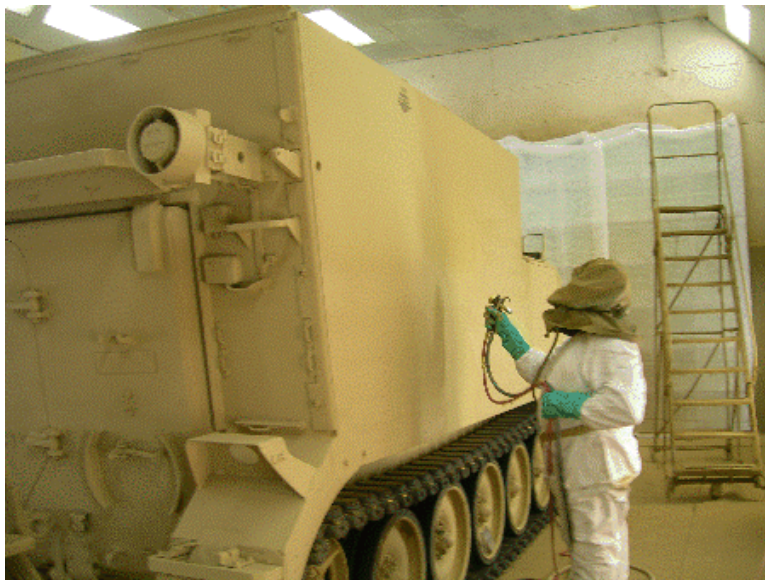
Figure 12. Painter applying Hentzen Coatings MIL-C-53039 coating using the DUX spray gun.
